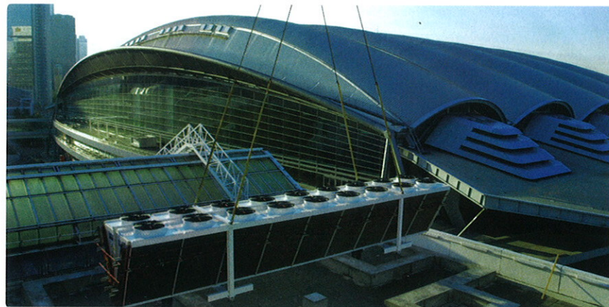
The LU-VE EHL dry coolers are lifted one by one on to the roof of Hall 4 by crane – in the background modern Hall 3.
