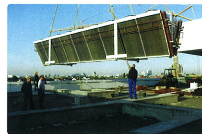
New foundations had to be prepared for the new dry cooler on hall Level 4.3.
