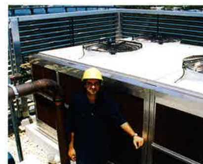
James Aye from AMZ Engineering with AIRA Pre-Cooler in front of Lu-Ve SHLT361A 250 kW Dry Cooler unit
