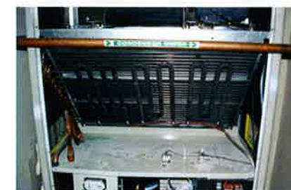
One of the apartment 30 kW water cooler package units
