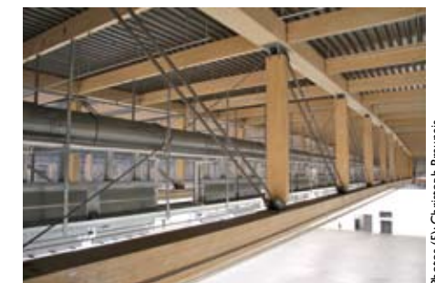
A total of 288 one- and two-sided induction devices are used to circulate the air around the hall
