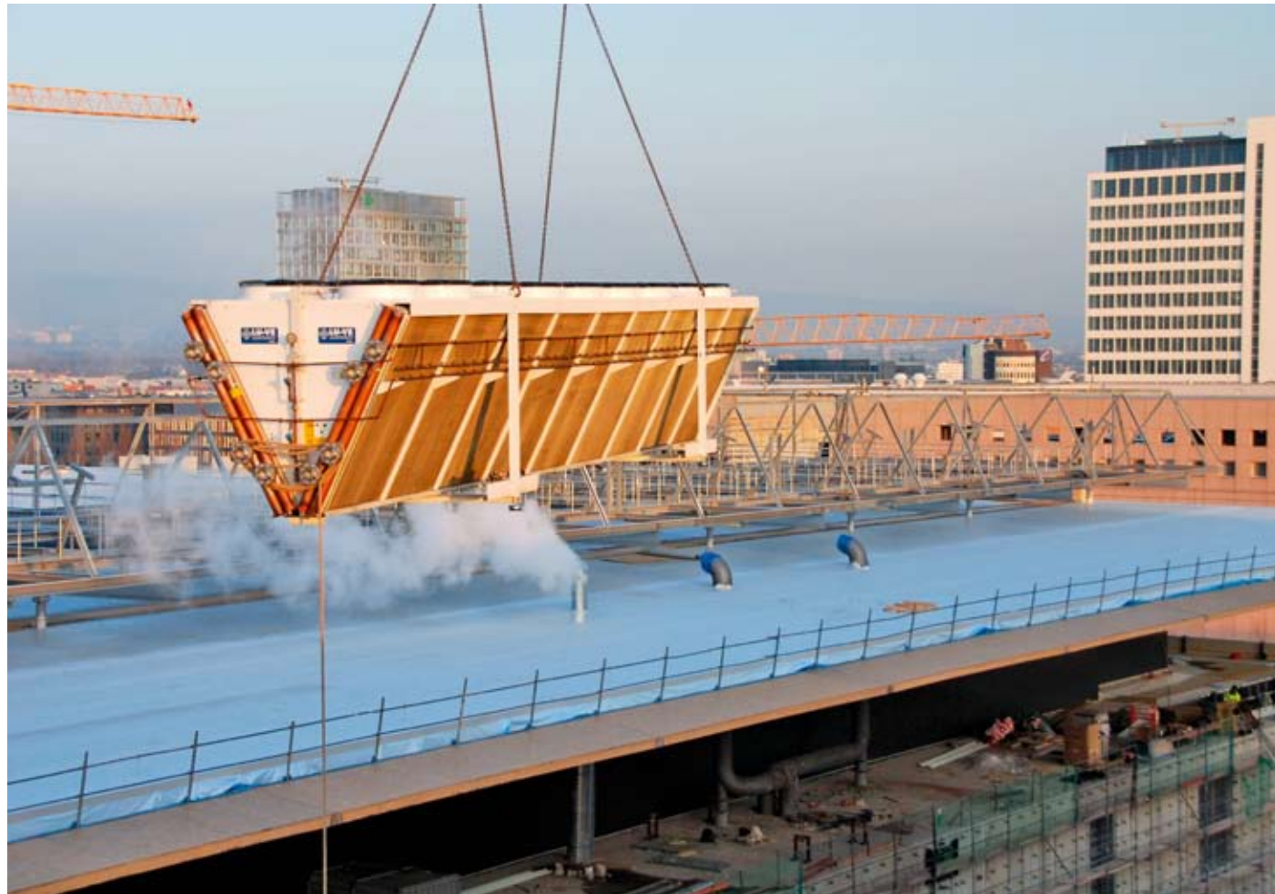
One of the 16 recooling units is lifted onto the roof of Hall 11
