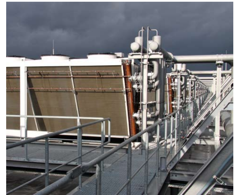
16 1.5 MW Lu-Ve Contardo recooling units adorn the roof of Hall 11
