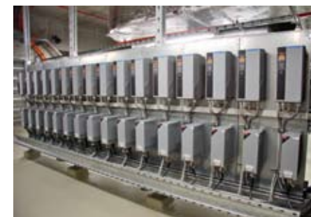
Each of the 16 recooling units has two frequency converters to control speed
