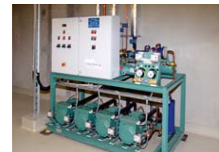
Combination system for normal refrigeration and deep freezing for a café
