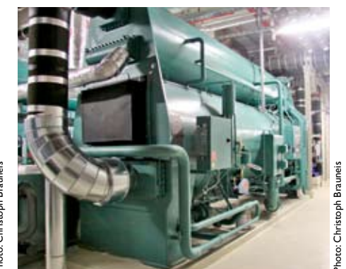
Absorption refrigeration machines with a refrigeration capacity of 2.8 MW
