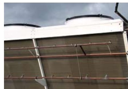
Recooler spray mode is only triggered when external temperatures rise above a set level
