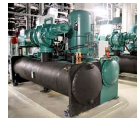
Two rotary screw compressors with a refrigeration capacity of 1.2 MW each
