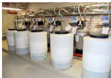
Water treatment for recooling spray mode
