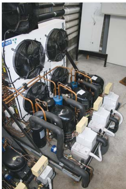
The larger unit, using the three LU-VE STFV370 condensers
