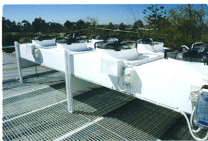
the eight fan LU-VE EHV 63 F condenser unit on the roof of the market
