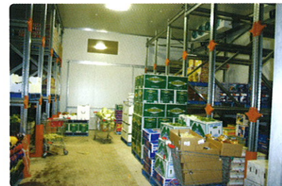
The large fresh food and produce storage coolroom with LU-VE S3HC 362E 50 Unit Coolers top right
