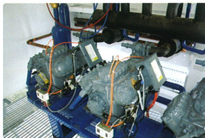
The medium temperature rack with Copeland Standard Reed Semi-Hermetic D6SL2-250 AWM/D Compressors
