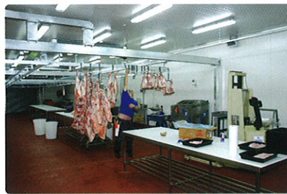
The large meat boning room has a LU-VE SHDS 368N32 evaporator which moves air up through its centre sending cold air out the sides and not directly onto staff below.
