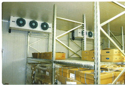
The beef coolroom with LU-VE SCH3272 E50 Unit Cooler evaporators
