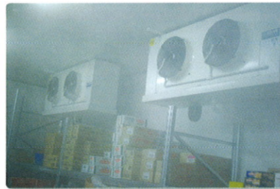
The freezer room with two LU-VE NHI 336 E4 Unit Coolers
