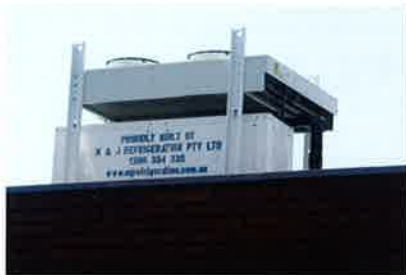
The plug and play refrigeration system in a box on the roof of the supermarket
