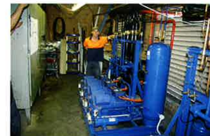
Simon Warde with the Bock high temperature compressor racks
