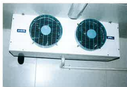
LU-VE BHC-SHC Unit Cooler evaporators
