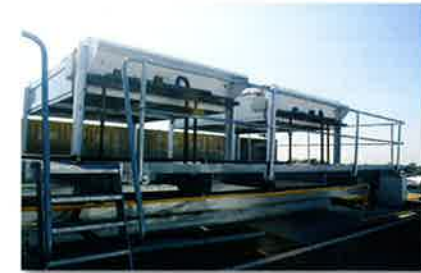
SHVN 305 with 284 kW capacity and an SHVN 264 with 264 kW capacity
